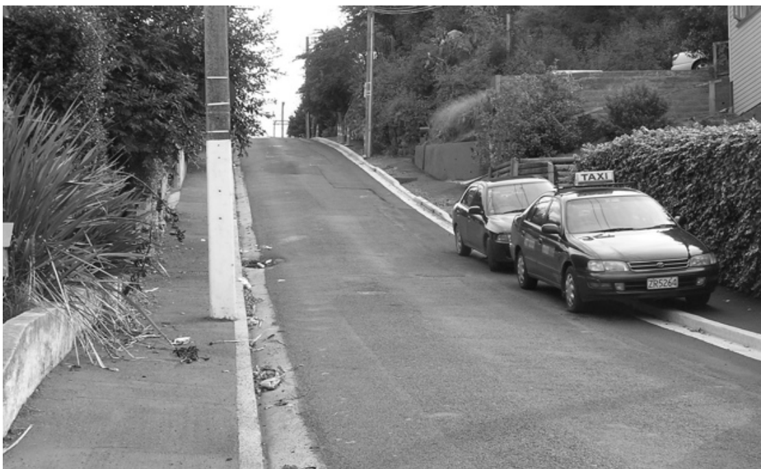
Figure 5: Ventnor St, The “available” footpath. In current “Parking on footpath” streets, care must be taken to see that the remaining usable footpaths are kept clear of obstructions, with consideration given to putting electricity and phone wiring underground to increase the width of the footpath. (In practice, most people seem to walk on the road in this street, because of the obstructions on both footpaths.)
