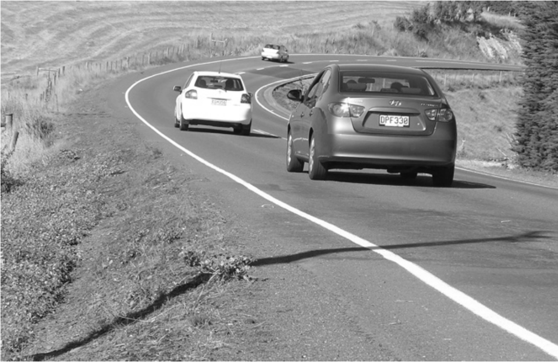
Figure 2. A closer view of the corner they were walking, showing narrow verge, uneven surface and steep unstable slope.
